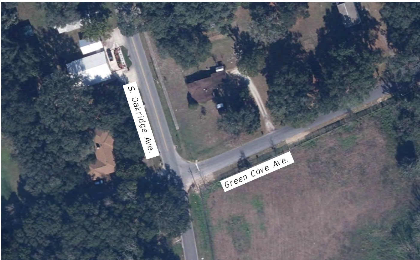
S. Oakridge Avenue at Green Cove Avenue
